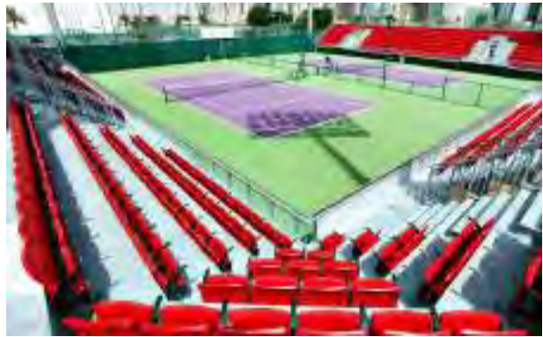
Refurbishment of Khalifa Tennis & Squash Complex [QATAR OLYMPIC COMMITTEE]
