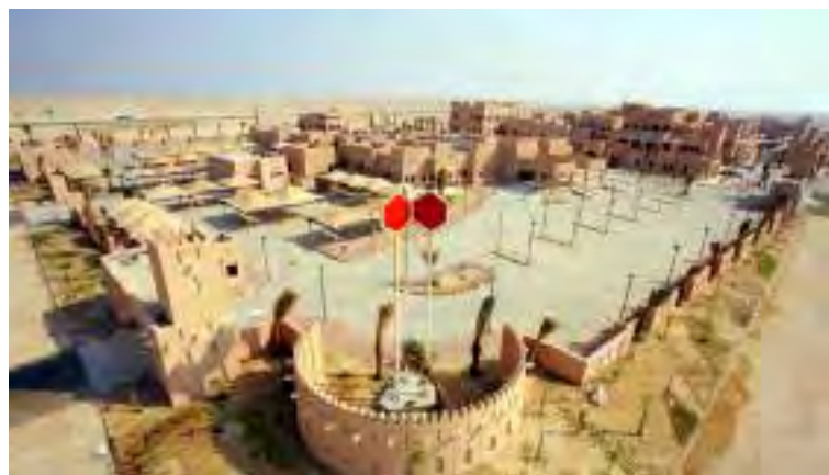
Public Services Complex at Al Dhaayen [ASHGHAL]
