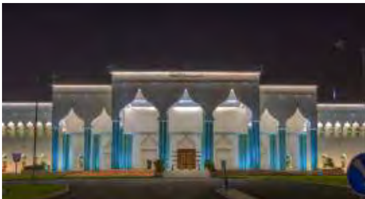
Refurbishment of Amiri Diwan – Phase II [PEO]
